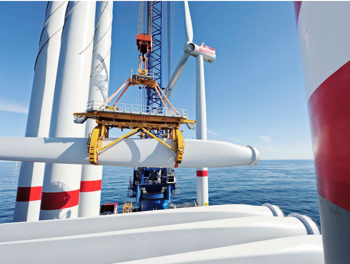
↑ Offshore wind farm construction in progress in the North Sea, Germany.
